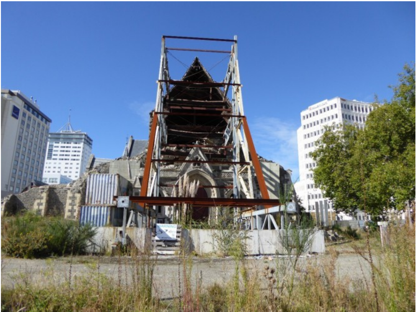
Christchurch Cathedral destroyed by earthquake
